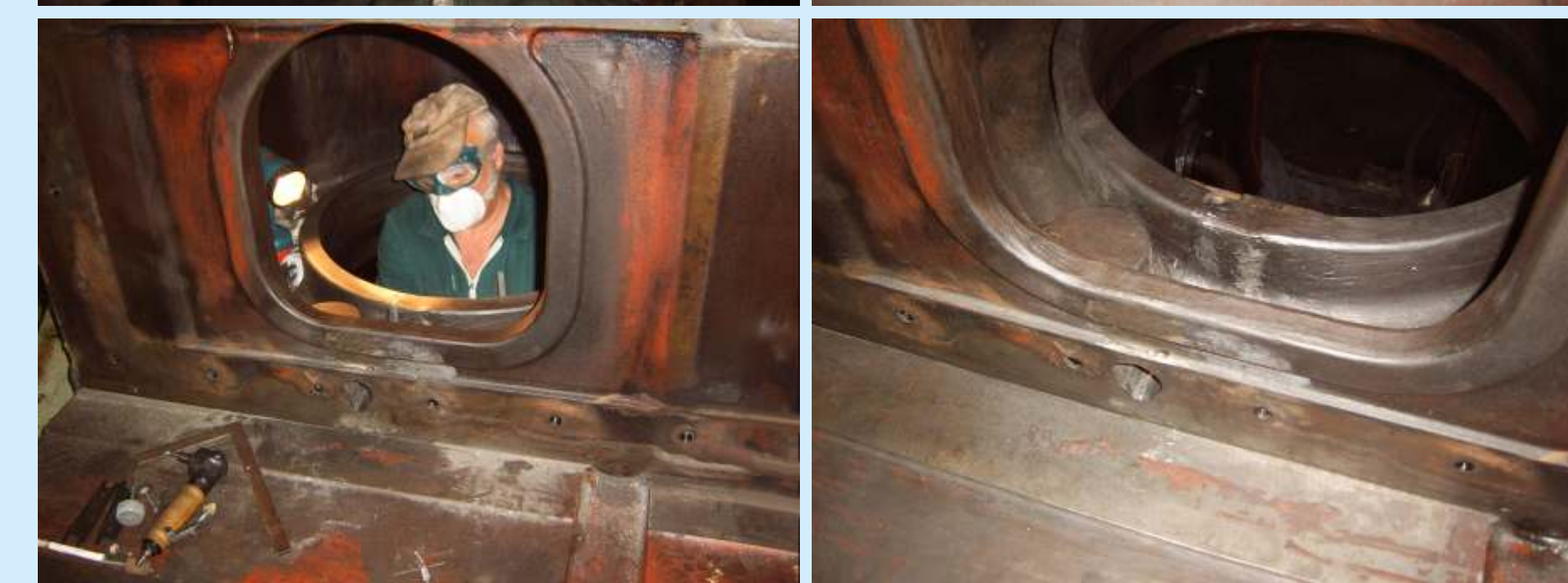
Final touches of machining on the reconstructed body after the crack repair (fig.7 and 8)
