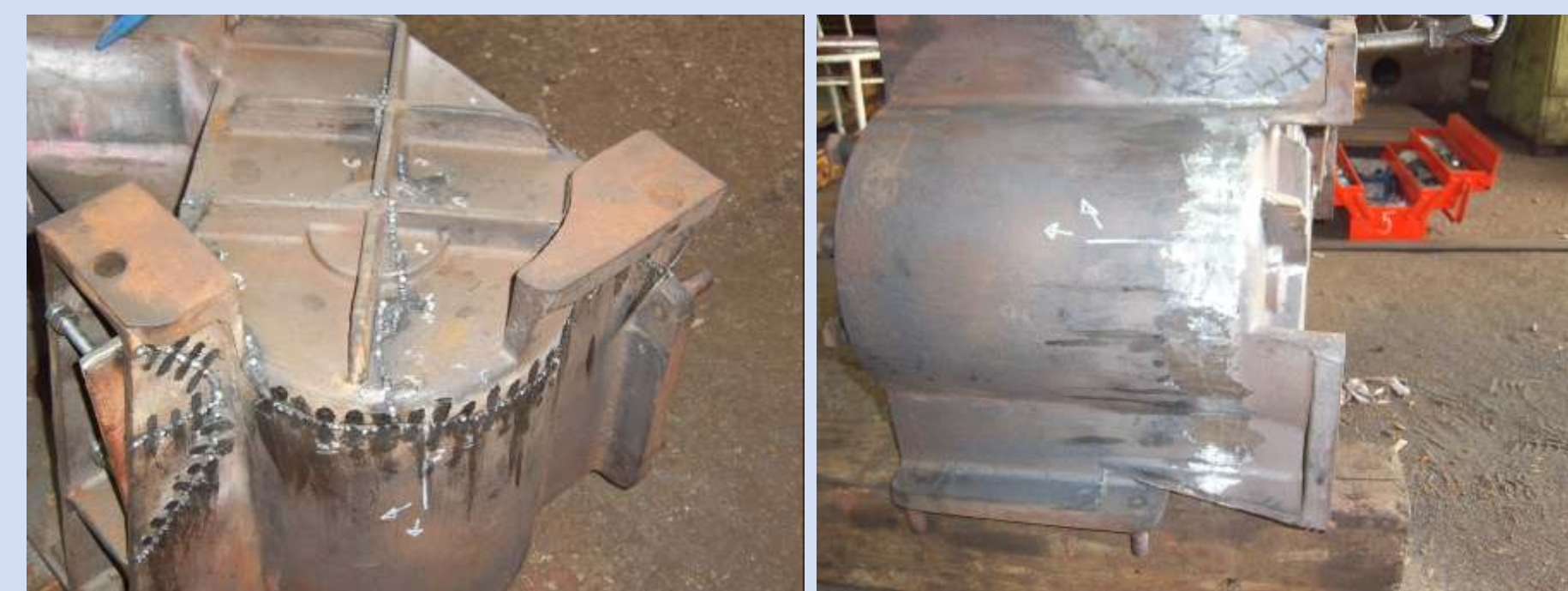
Moment of the Metallock repair of the piston pump casing (fig. 5)
