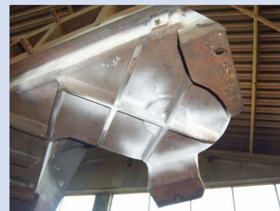
Test for repair quality (fig.7)
