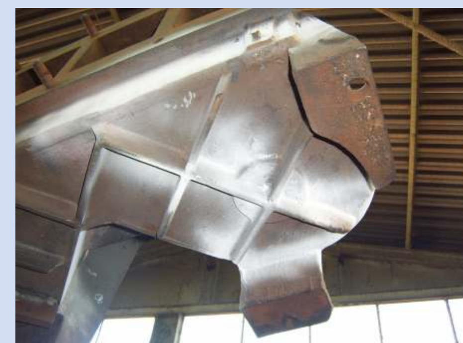
Test for repair quality (fig.7)
