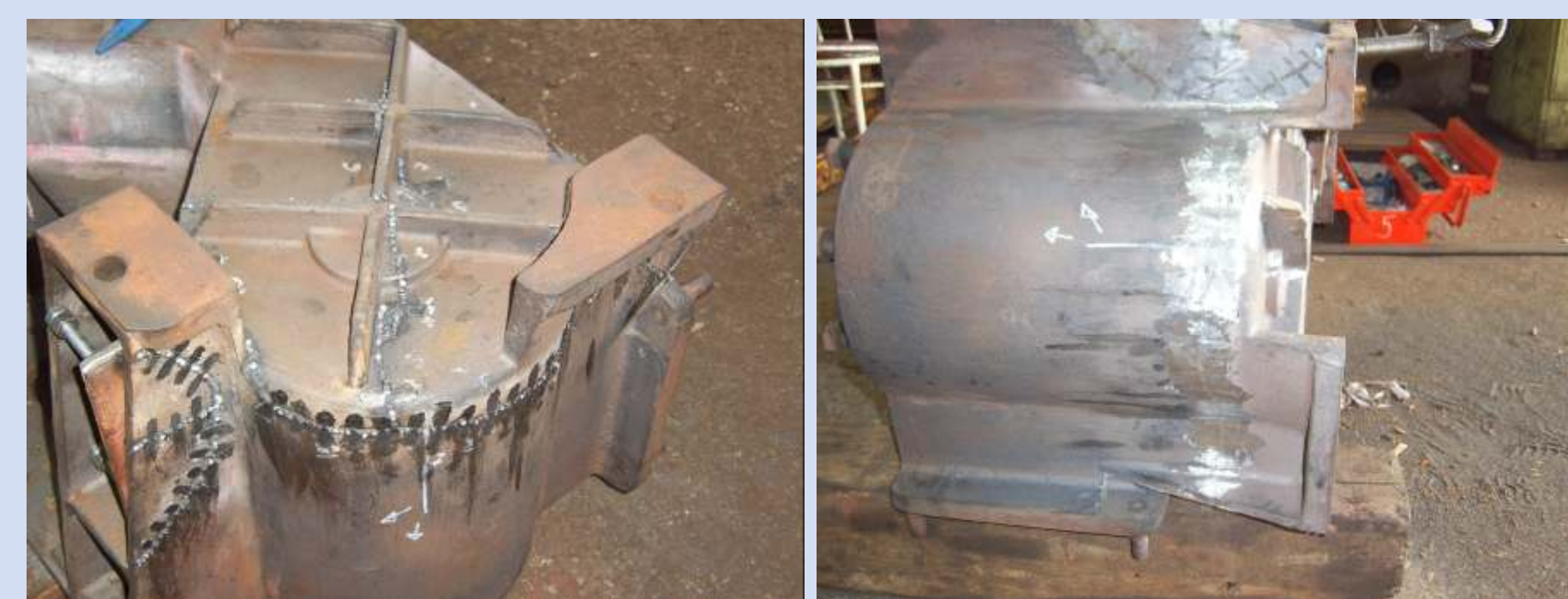
Moment of the Metallock repair of the piston pump casing (fig. 5)
